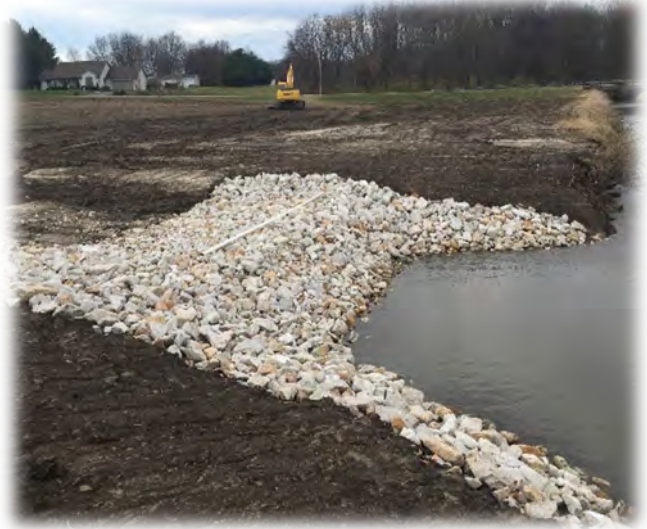
Grade Control Structure – Block Chute
